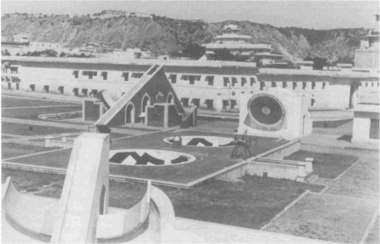
FIG. 16.23. JAIPUR OBSERVATORY. This photograph, taken from atop the Samraṭ Yantra within the Jaipur observatory built by Jai Singh, shows several of its giant masonry instruments. The Samraṭ Yantra, a triangular gnomon, has a height of nearly 90 feet, above the ground and a base of 147 feet. The corresponding instrument at Delhi is substantially smaller (60 feet, 4 inches high). The two complementary concave hemispheres of the Jai Prakāṣa (17 feet, 10 inches in diameter) appear in the
