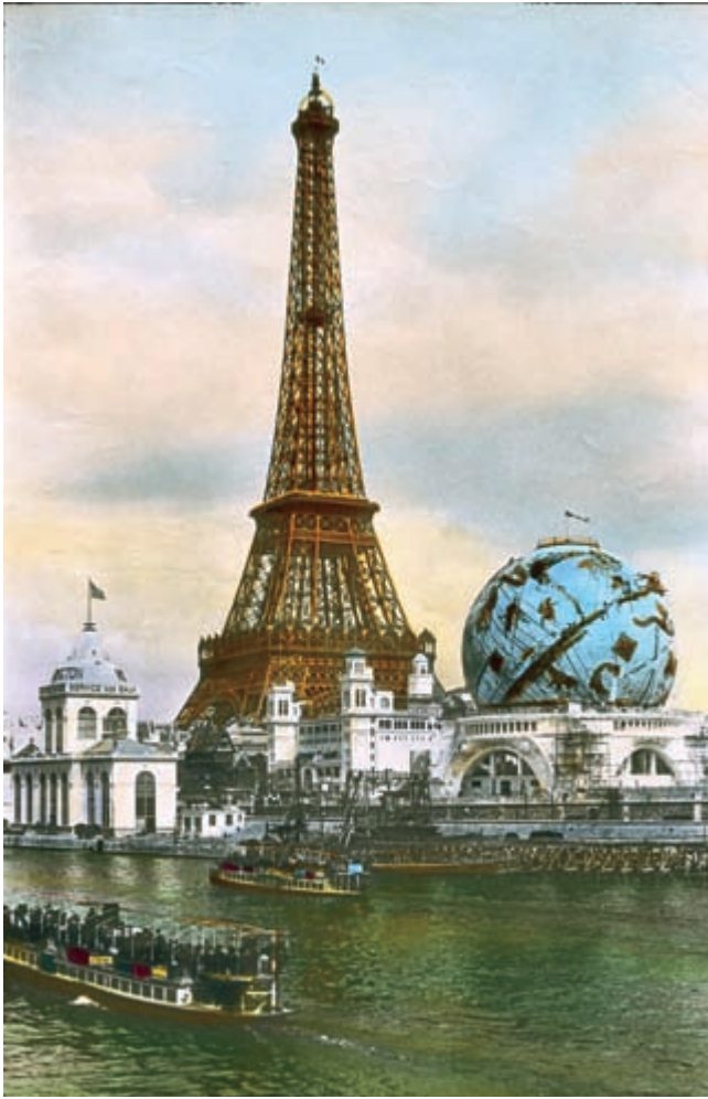
FIG. 341. LE GRAND GLOBE CÉLESTE AT THE EXPOSITION UNIVERSELLE IN PARIS, 1900. The huge celestial globe had a diameter of 46 meters and rested on a construction of four masonry piers. Inside it was a second celestial globe with a diameter of 36 meters, and within that globe was a terrestrial globe with a diameter of 8 meters. Visitors could pay an additional fee and, using a spiral staircase in the terrestrial globe, climb up to the North Pole and look at the sky, which was painted on the inside of the second celestial globe. Image courtesy of the Brooklyn Museum Archives, Goodyear Archival Collection.
