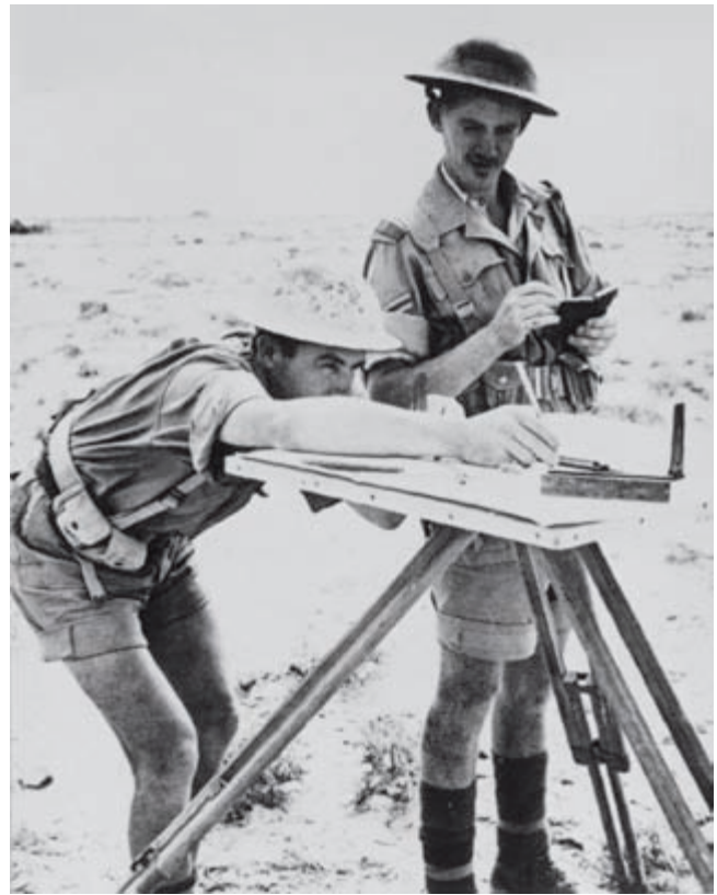
FIG. 541. BRITISH MILITARY SURVEYORS PLANE TABLE IN THE WESTERN DESERT IN WORLD WAR II. Although aerial photography was by then widely used for mapping behind enemy lines, plane tabling was still used for mapping of British rear areas. Image courtesy of Defence Surveyors’ Association, U.K.
